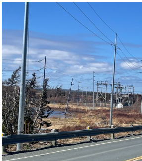
Relocation of 24L in St. John's out of water supply.
