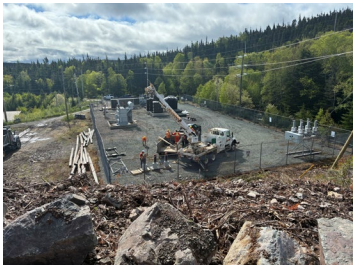
Early site work at Lockston Substation in Bonavista area.
