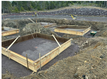
Foundation construction at Summerville Substation in the Bonavista area.
